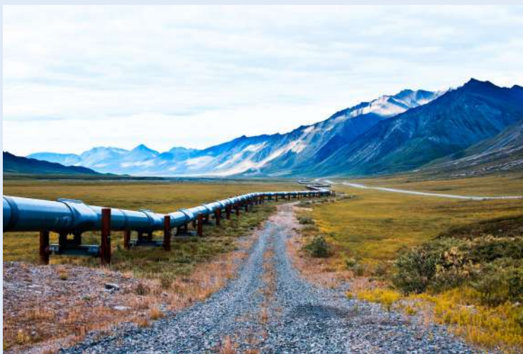
Figure 2.2: This oil pipeline passes very close to a national wildlife refuge.
