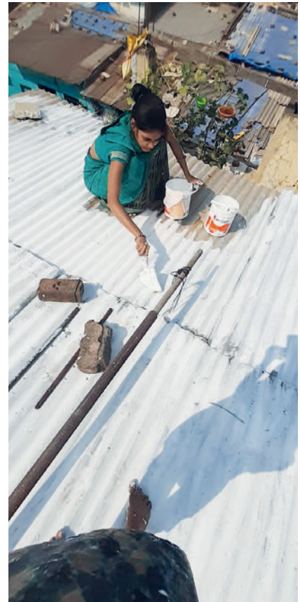
Figure 2: A woman in Ahmedabad painting her home roof with solar reflective paint (Credit: Mahila Housing Trust)
