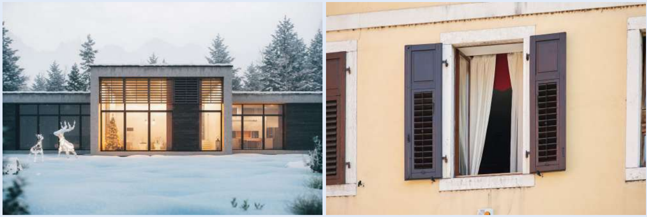
Figure 33: Large, sealed windows that let in sunlight (left) for passive heating and windows open for ventilation (right) for passive cooling.
