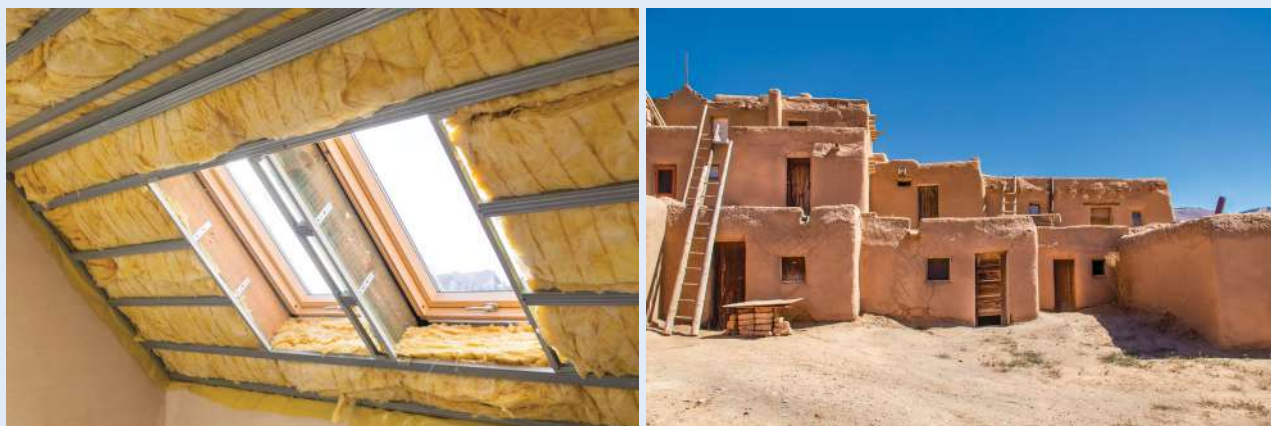
Figure 32: Wall insulation (left) for passive heating and clay walls (right) for passive cooling.
